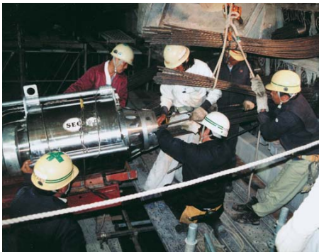
Fig. 17: TENSAM 9750 kN stressing jack (37 x 0.6") operating in Japan
