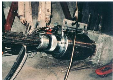
Fig. 22: TENSAM 4800 kN stressing jack used for stressing 19 x 0.6" anchors
